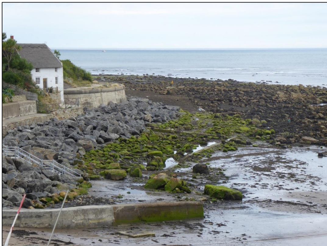
Figure 2.1. Location of new granite rock armour at the foot of the seawall, note the green (colonised) natural boulders which have been placed in front of the granite rock (August 2018).
