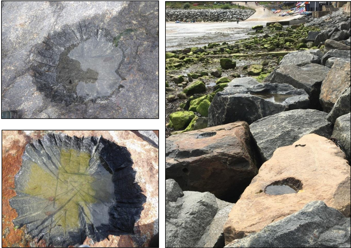
Figure 2.2. Examples of saw cut artificial rock pools roughly 300 mm diameter x 150 mm deep.
